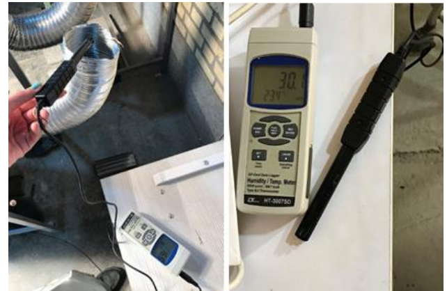
Figure 4. Measure the outlet temperature of the device with a thermometer
